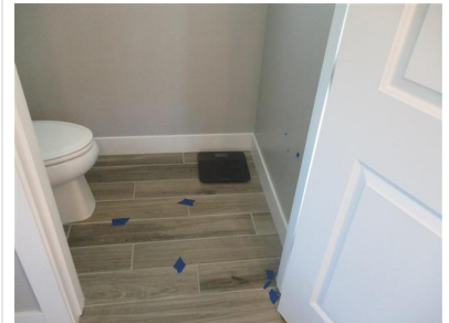
7.1 Item 5 (Picture) master toilet closet
